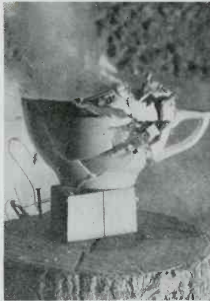
These two photographs were made by Arthur Palme, Pittsfield, Mass., with a home-made variation of the Speedlight originally developed by Professor Harold E. Edgerton of MIT. In both cases the damage was done with a 22 cal. rifle, the lamp bulb photo being made at 1/15,000th second and the teacup at 1/10,000th second
