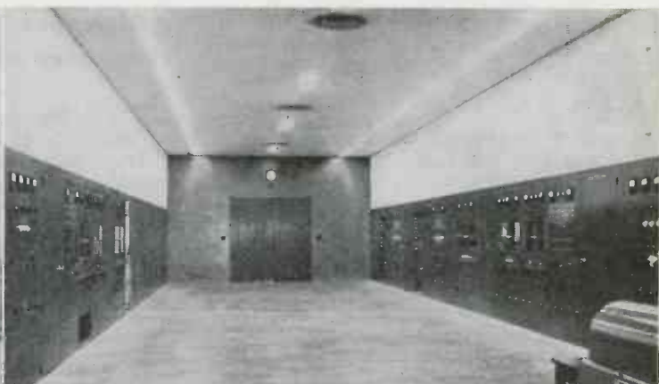
General view of the OWI-CBS international shortwave transmitter building, and a glimpse down the transmitter room each side of which provides space for a complete 200kw transmitter. Left, rear view of the modulator which delivers an output of 150 kw audio power
