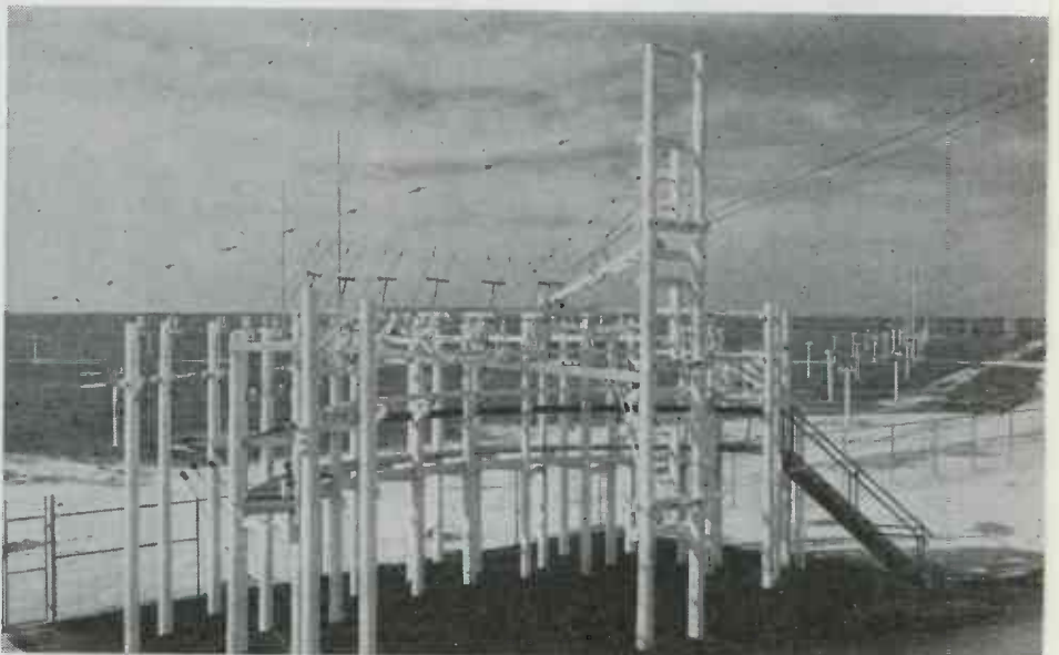
The elaborate antenna switching system designed to facilitate the selection of any of the directional antennas and coupling them to the two 50 kw and the 200 kw transmitter
